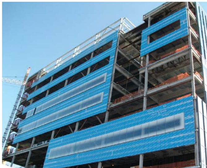
Curved & Straight Panels assembled with Densglass sheathing and Blueskin SA.
